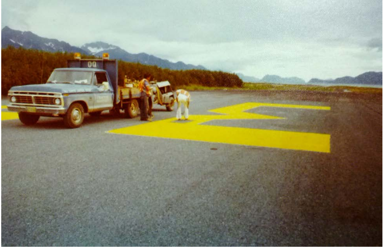
Figure 18: July 21, 1975, work crew painting '33' on runway 15-33 (today's 16-34). Photo from DOT&PF archives.
