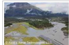
Seward Airport Improvement Project (#54857)
