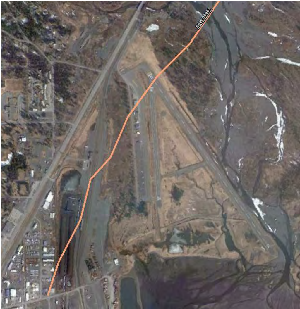
Figure 7. Aerial photograph from 2011 showing the AHRS location of SEW-00007 in relation to the Seward airport and the Alaska Railroad Yard.
