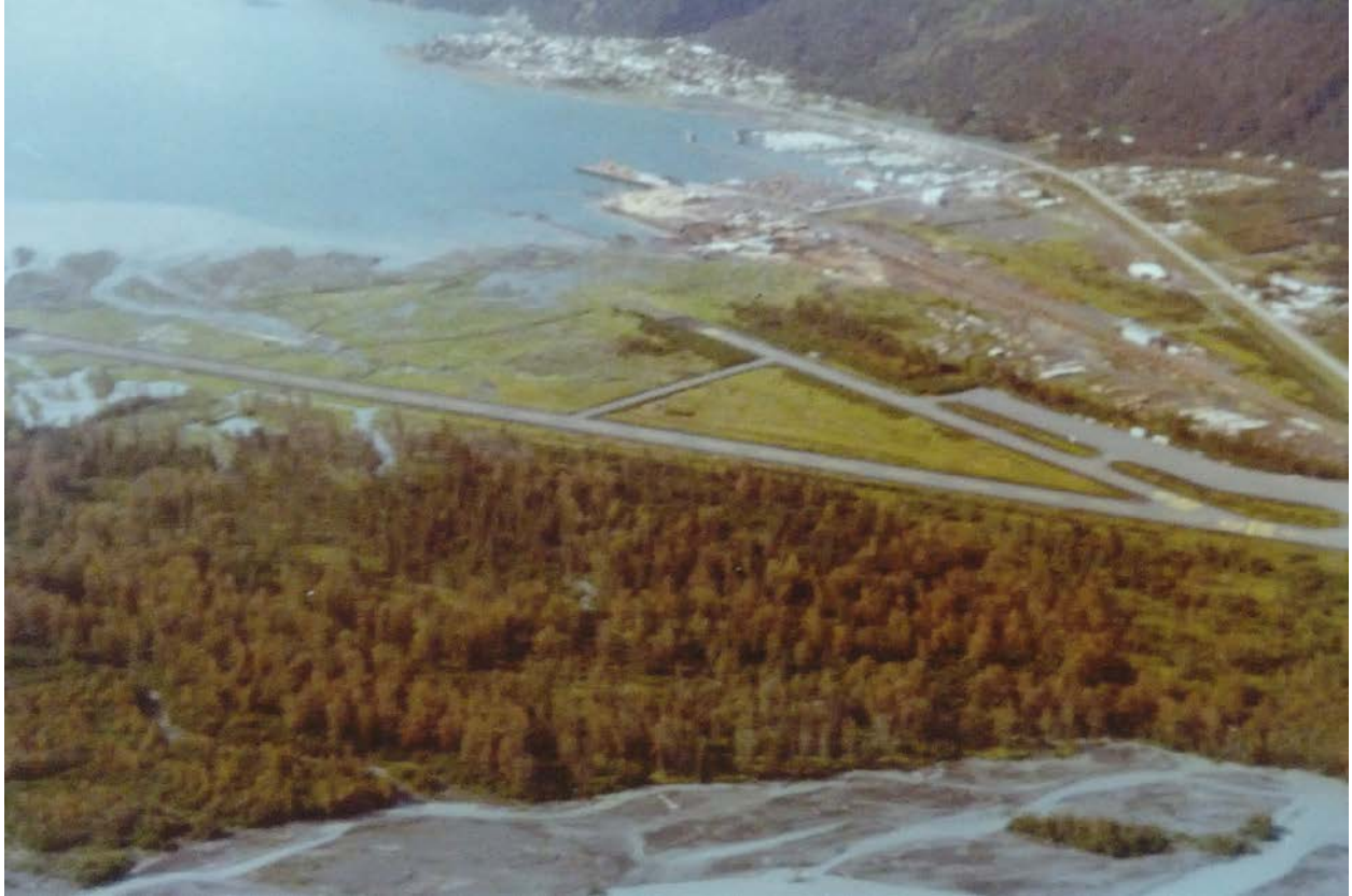
Figure 19: July 1975, Overview of Seward Airport after runways, taxiways, and apron being surfaced with bituminous sealcoat. Photo from DOT&PF archives.
