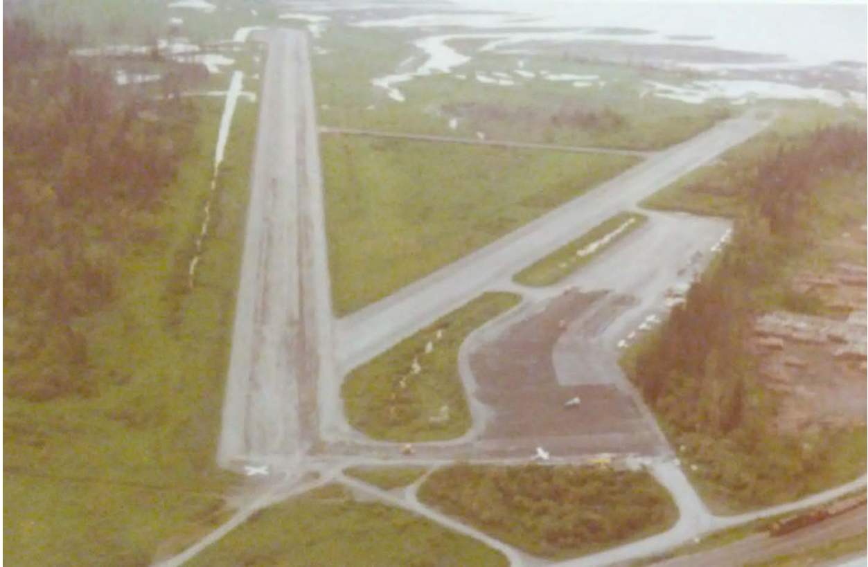
Figure 16: July 8, 1975, Overview of Seward Airport prior to runways, taxiways, and apron being surfaced with bituminous sealcoat. Photo from DOT&PF archives.
