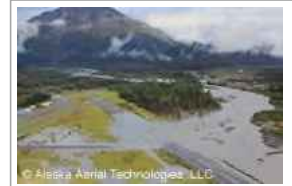
Seward Airport Improvement Project (#54857)
