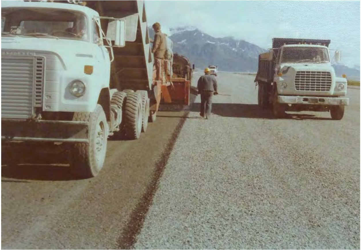
Figure 17: July 1975, top course seal operation in progress. Photo from DOT&PF archives.
