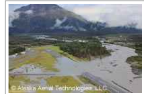
Seward Airport Improvement Project (#54857)
