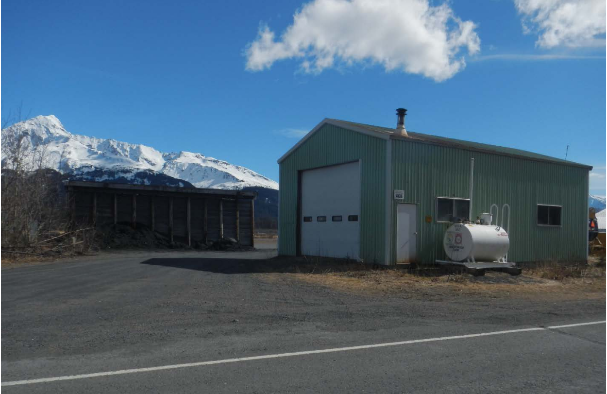
Figure 23. April 20, 2017 Photo of Seward airport SREB and sand shed.
