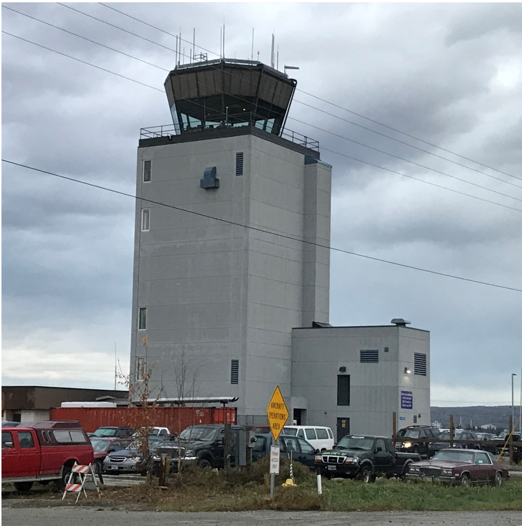
Photo 2-17. Air Traffic Control Tower on the East Ramp
