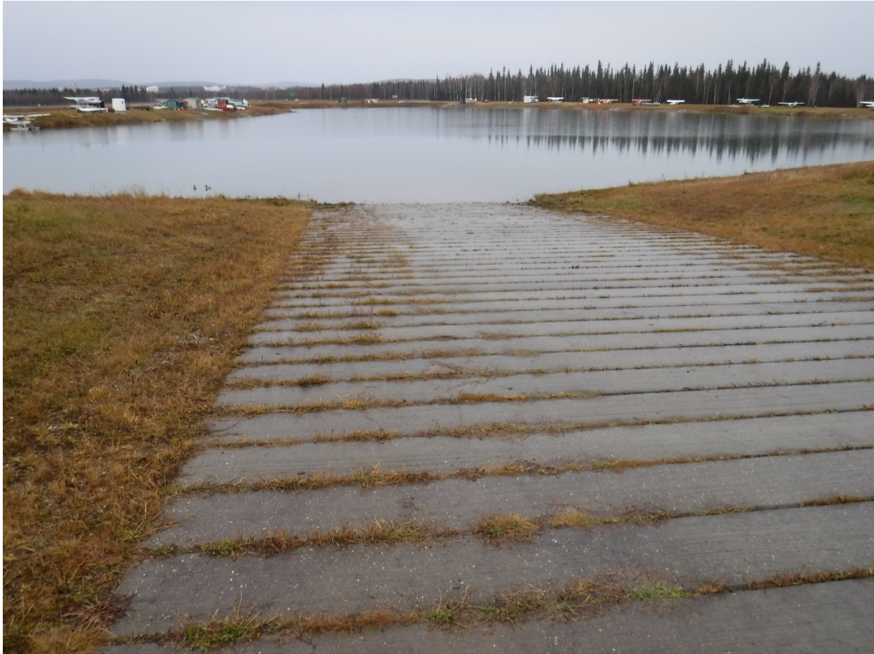
Photo 2-8. Floatplane Ramp at Floatpond Extension
