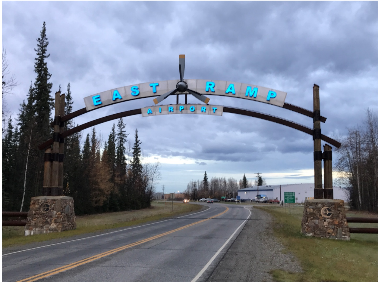
Photo 2-10. Sign at Eastside Entrance
