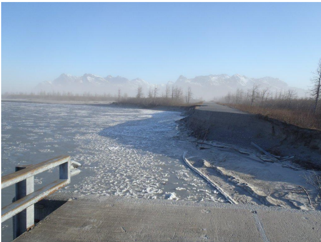
Figure 1 – Bridge 339 looking south August 14, 2012
