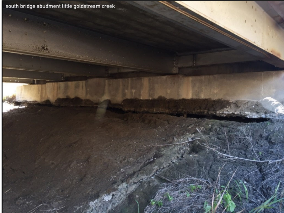
Photo 3-12 Little Goldstream Creek Bridge No. 678 South Bridge Abutment
