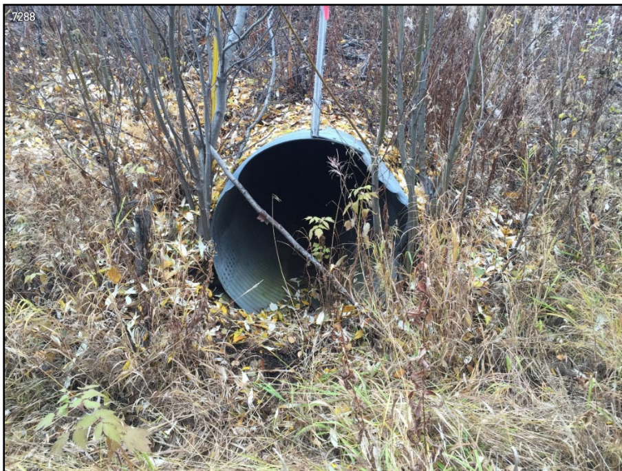
Photo 3-7 Parks Highway MP 312.6 48-in culvert inlet, northbound side of road
