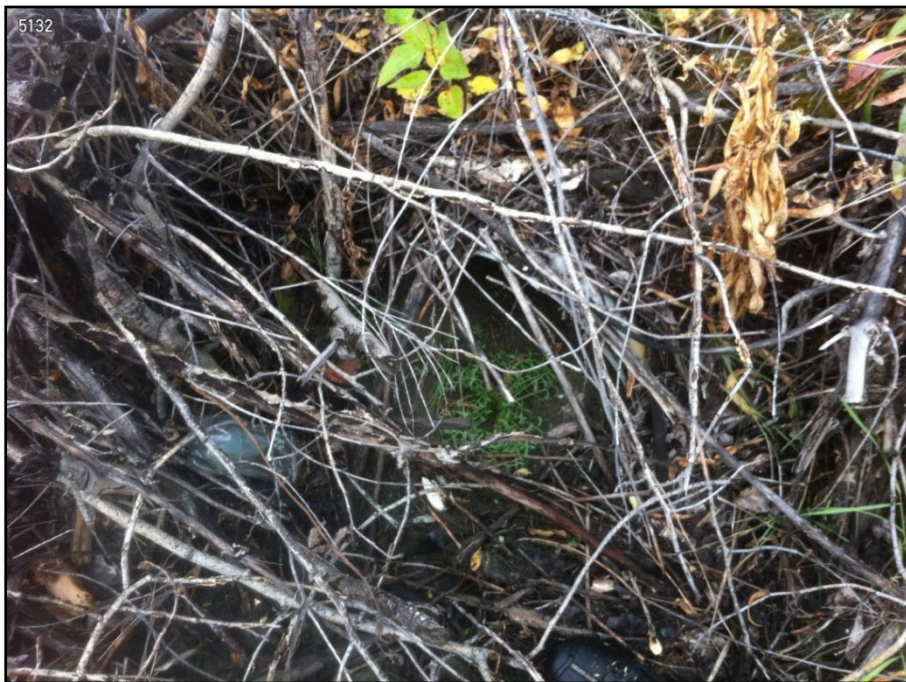
Photo 3-3 Parks Highway MP 305.5 18-in culvert outlet, southbound side of road
