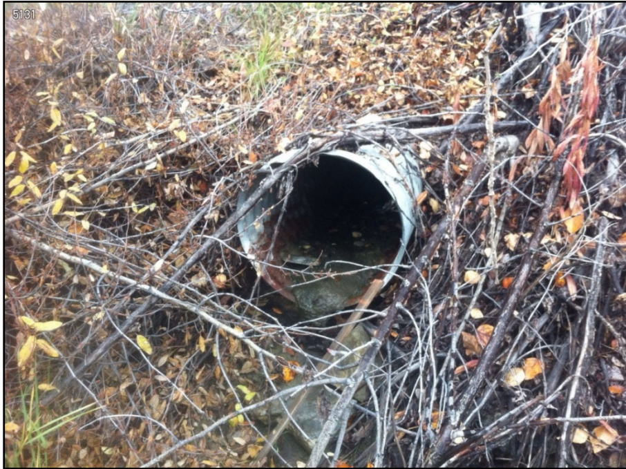
Photo 3-2 Parks Highway MP 305.4 18-in culvert outlet, southbound side of road
