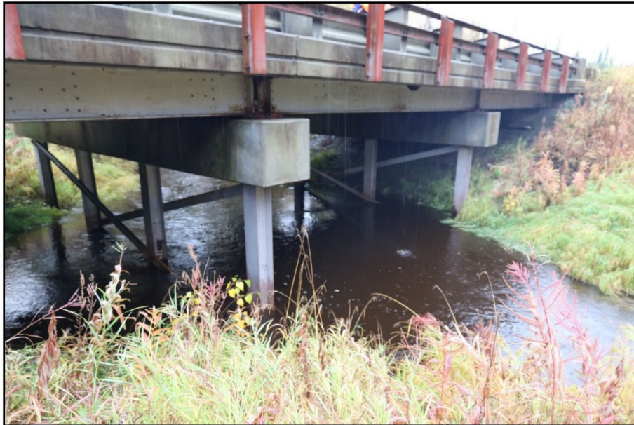
Photo 3-10 Little Goldstream Creek Bridge No. 678, looking downstream (Northwest)
