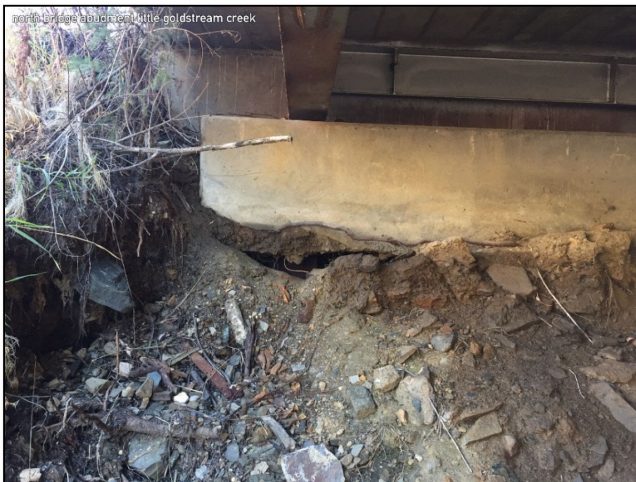
Photo 3-11 Little Goldstream Creek Bridge No. 678 North Bridge Abutment
