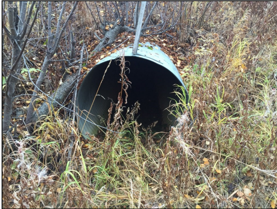
Photo 3-8 Parks Highway MP 312.6 48-in culvert outlet, southbound side of road
