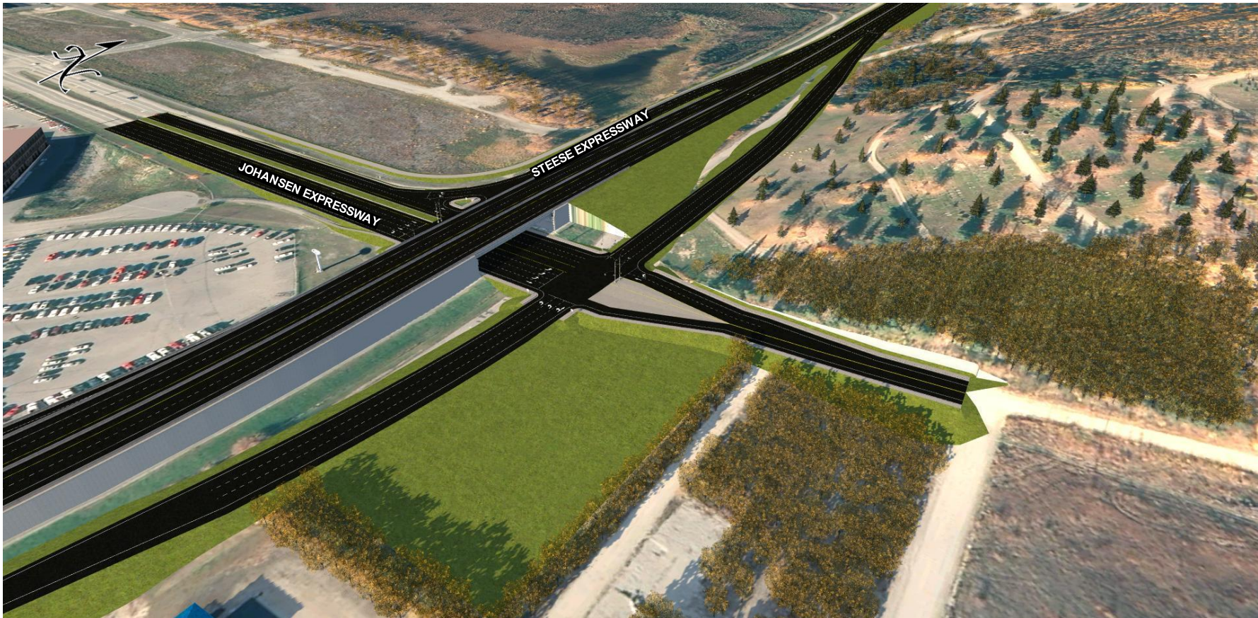
Figure 3.2: Tight Diamond Interchange
