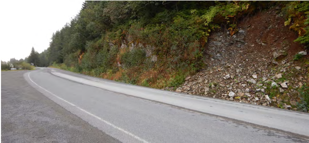
Figure 2: Miniature rock slide (right) as an example of ditch infill. (source: DOT&PF file photo, Point Whitshed Road MP ~0.6, 2019)
