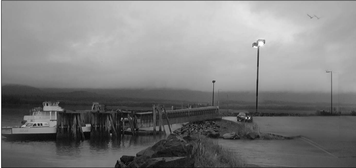
Alternative G3 ferry from the north parking area adjacent to Plaza Port West, looking northwest toward Gravina Island (Key View 5).
