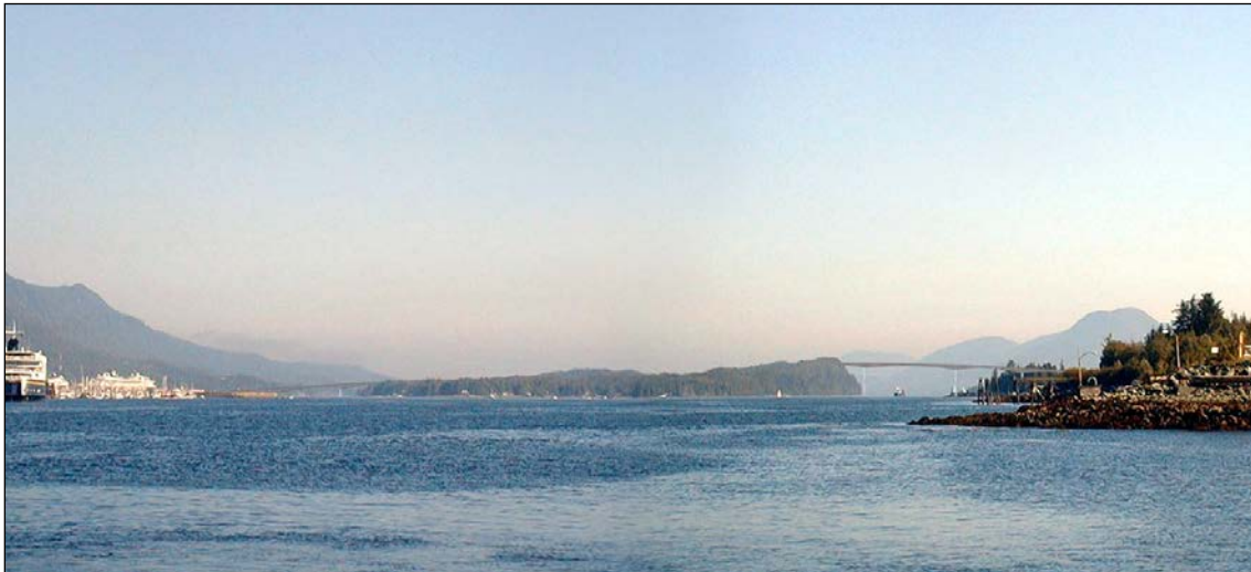
Alternative F3 bridges and Pennock Island as simulated in a view from mid-Tongass Narrows near the airport, looking south (Key View 6).
