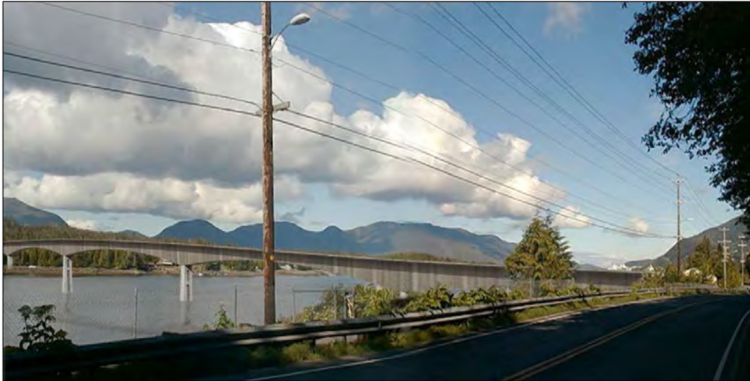
Alternative F3 bridge over East Channel as simulated in a view from South Tongass Highway south of the USCG Station, looking north (Key View 1).
