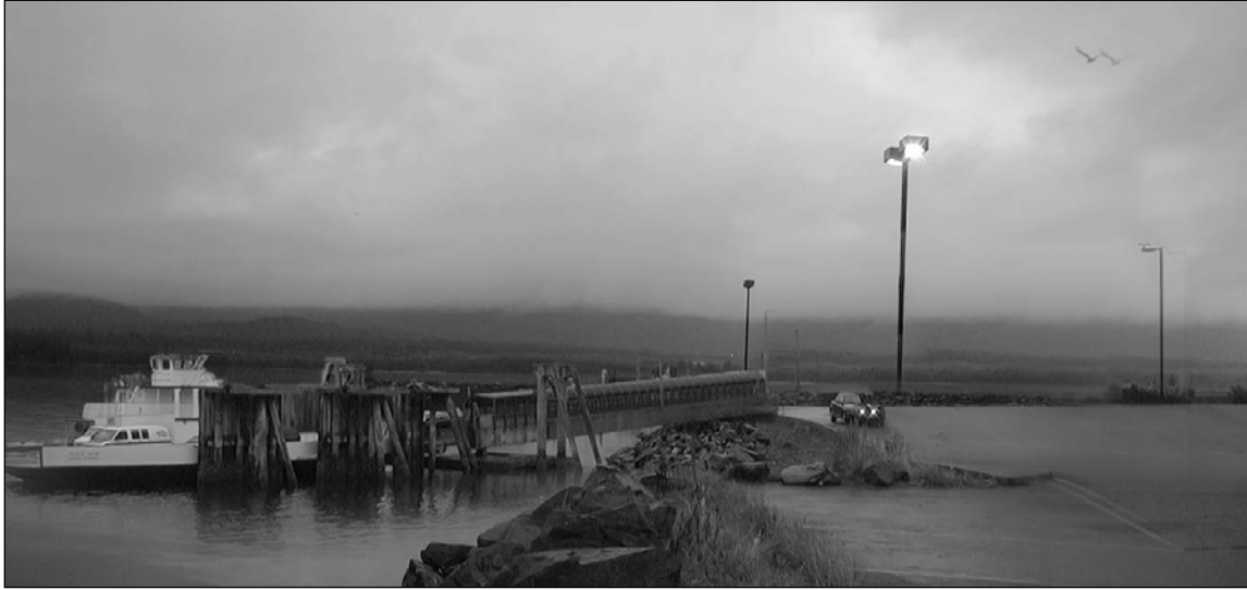
Alternative G3 ferry from the north parking area adjacent to Plaza Port West, looking northwest toward Gravina Island (Key View 5).
