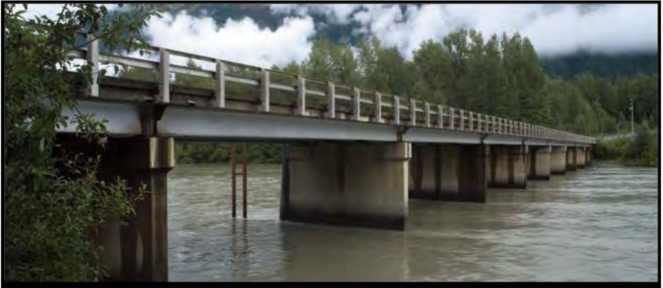
Photograph 1: Chilkat River Bridge
