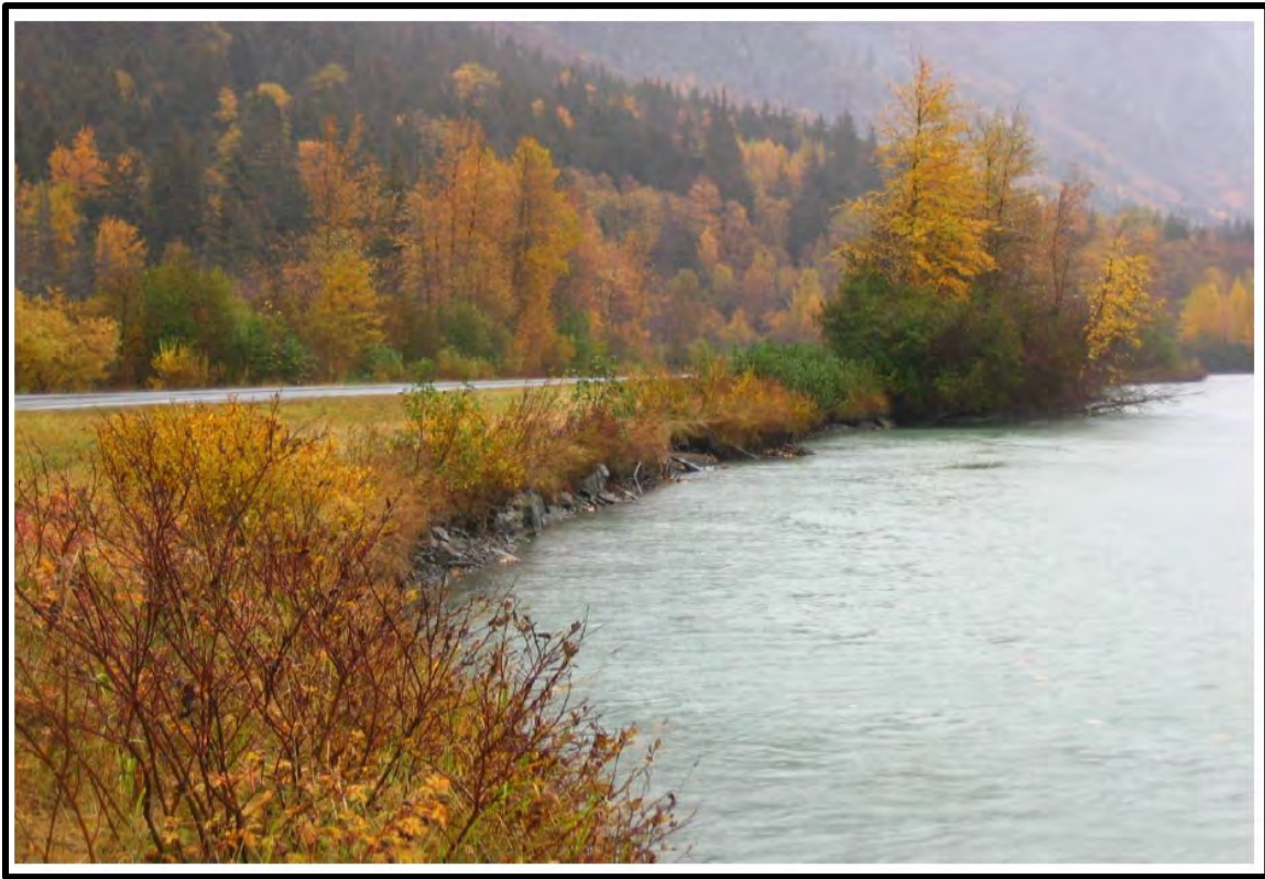
Photograph 4.21-5: Vegetated Riprap along the Bank of the Chilkat River
