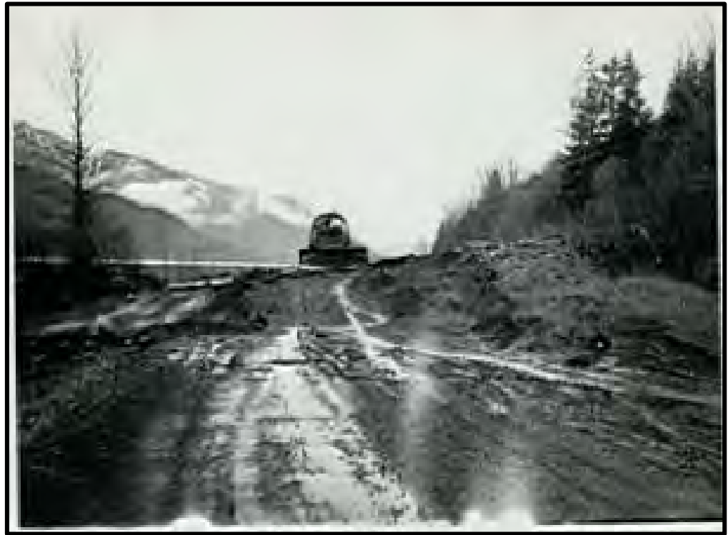
Photograph 4.21-4: Original Highway Construction “Loading Crushed at 25 mi”, circa 1949
