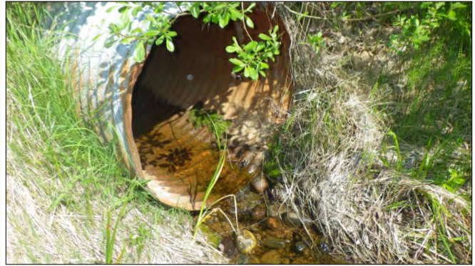
Figure 29.—MP 16.9 drainage, HH culvert outlet.
