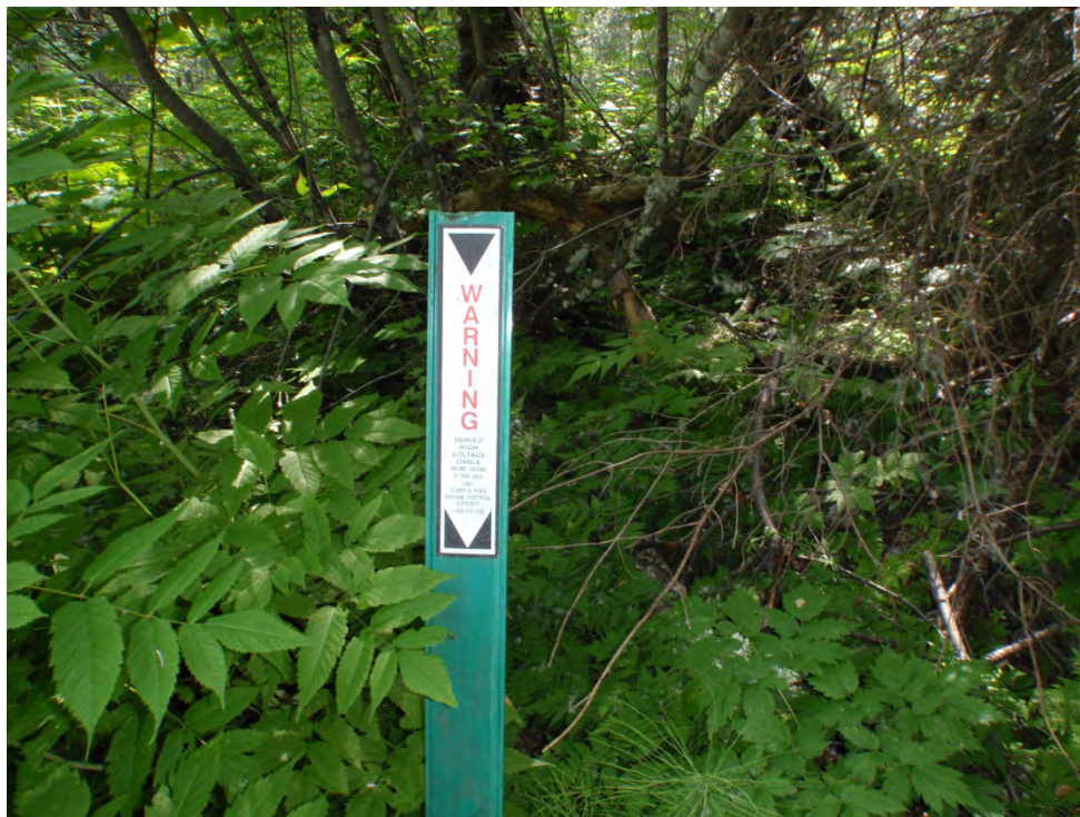
PMP 19.5 – Marker Identifying Power/Phone Line (believed to inside the HFP) (Photo Taken from near the Haines Highway – Looking West)
