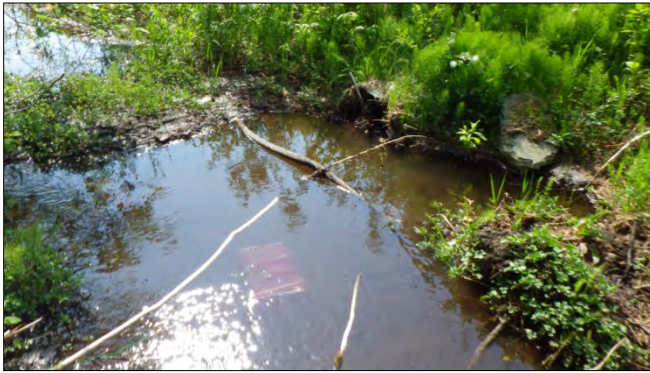
Figure 7.–HH culvert (FP7) inlet pond.
