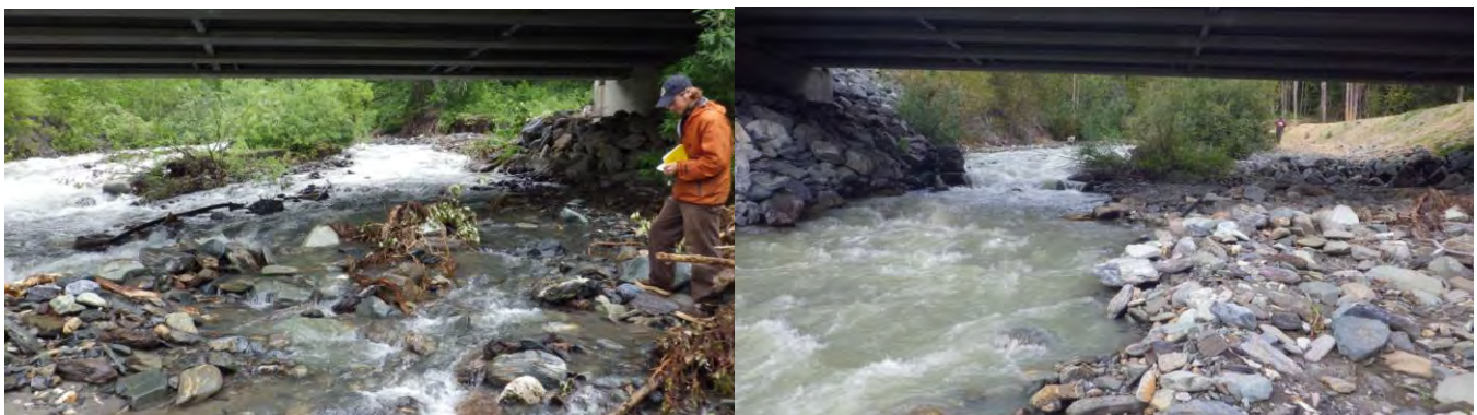
Figures 9 & 10. Left: Looking upstream from below Little Boulder Creek bridge before the launch apron raised the elevation in the overflow channel on river left (June 27, 2012). Right: Same view following embankment repairs with dry, elevated overflow channel (September 4, 2013).
