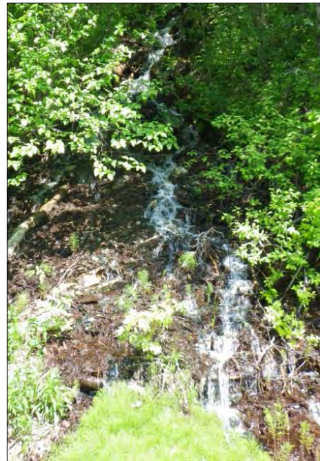
Figure 2.—Barrier falls on ditch at wpt 46.
