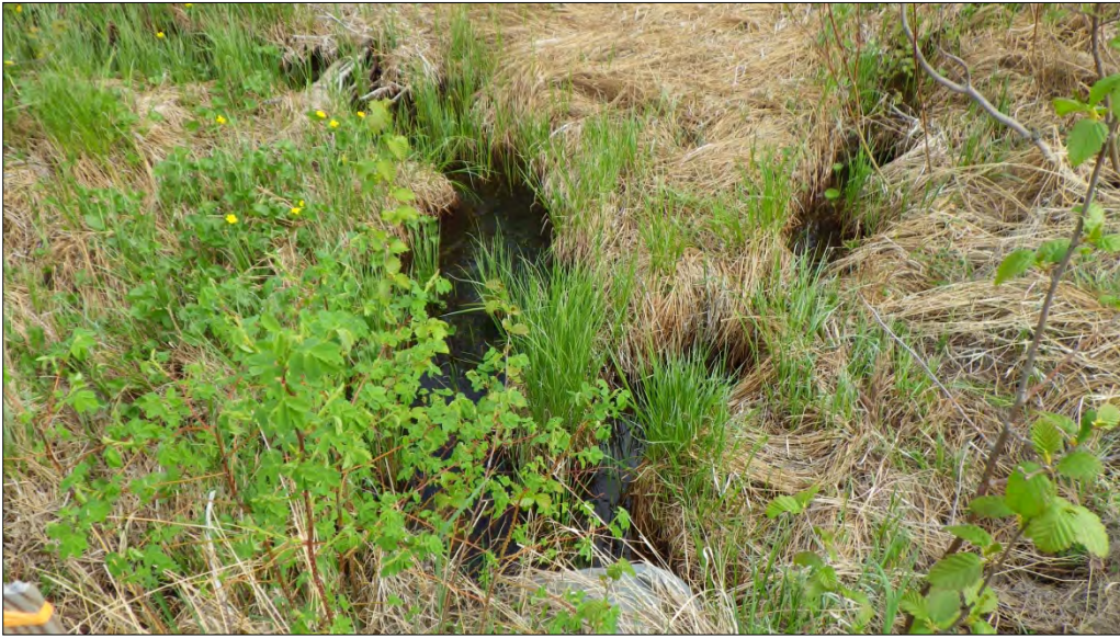
Figure 3.—Stream No. 115-32-10250-2006-3003 culvert (FP3) inlet.
