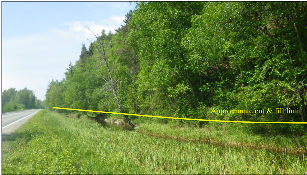
Figure 27.–MP15.0 ditch drainage falls adjacent to HH.
