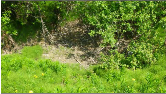
Figure 28.—MP 16.9 ditch drainage, upstream of HH.
