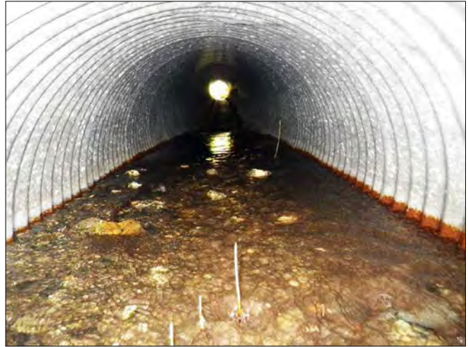
Figure 35.—Stream No. 115-32-10250-2070 culvert outlet, looking upstream. Photo courtesy of Matt Eisenman and Jim Latham, ADF&G Division of Sport Fish.
