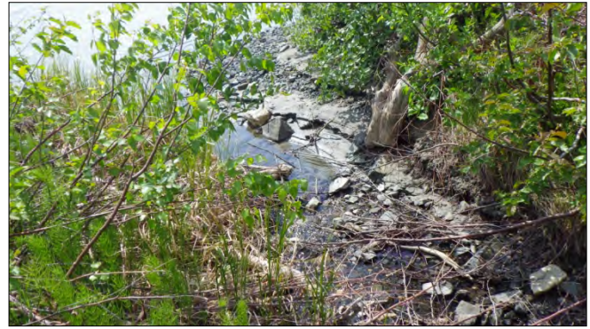
Figure 14.–Stream No. 115-32-10250-2022 downstream of HH culvert (FP11).
