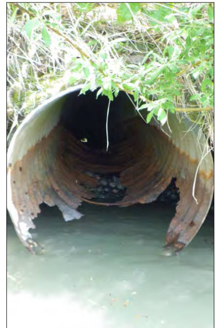
Figure 12.–HH culvert outlet (FP10).
