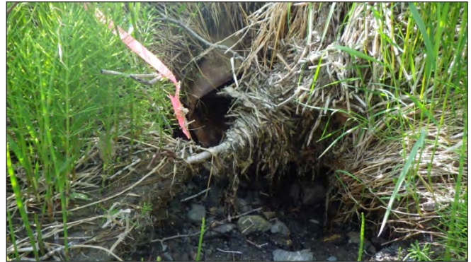
Figure 11.–HH culvert inlet (FP10).
