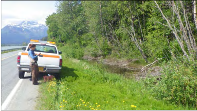
Figure 10.–Drainage upstream of HH culvert (FP10).
