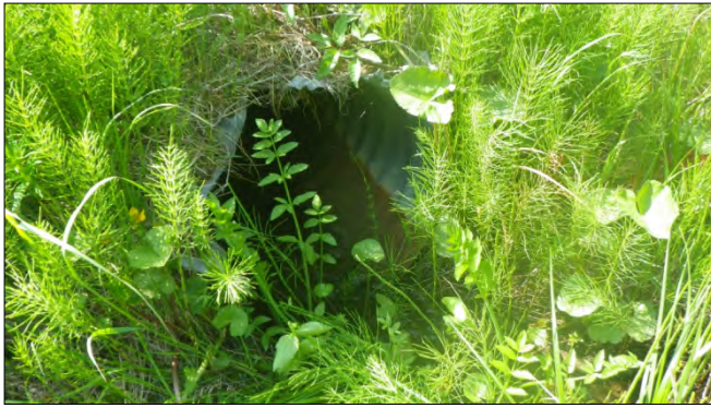
Figure 17.–Stream No. 115-32-10250-2030-0010 pond outlet, HH culvert (FP15) inlet.
