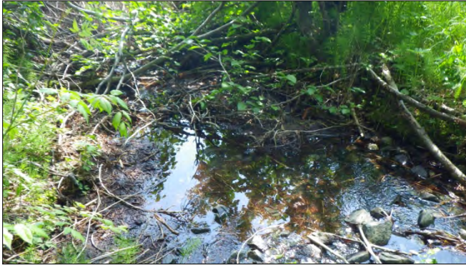
Figure 13.–Stream No. 115-32-10250-2022 upstream of HH culvert (FP11).
