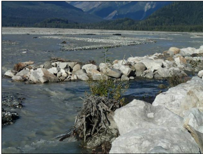
Figure 8. River training revetment (photo center) on the Klehini River closely resembles the configuration of a typical rock weir/spur structure proposed for the Haines Highway Project. Rock weirs/spurs would be larger and angled in the upstream direction. Note large boulders and woody debris in lower photo right. (ADOT&PF, August 2013).
