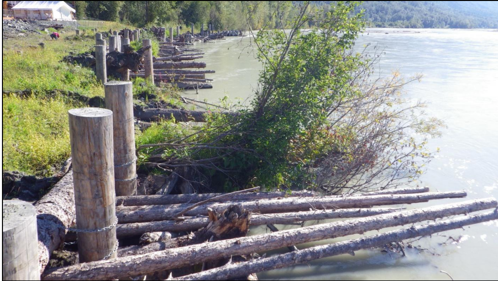
Figure 5. Klukwan wood revetment, looking downstream. (Courtesy ADF&G, 2013).
