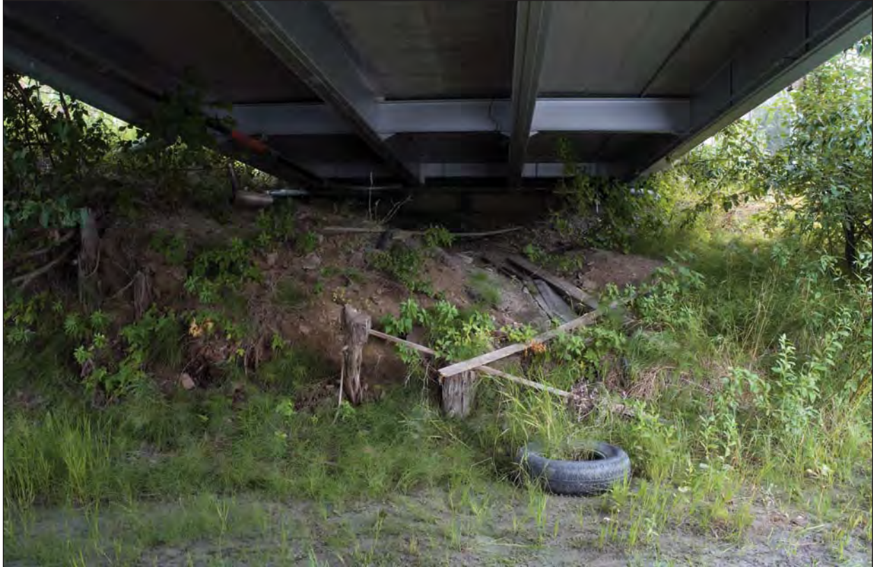
Figure H-10. Pilings from the 1943 bridge (SKG-549) in place beneath the southern end of the current bridge.
