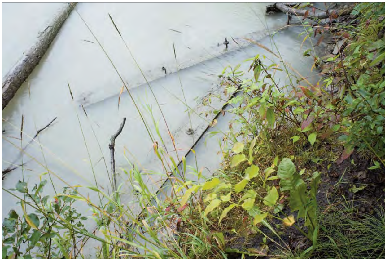
Figure H-7. Sway braces in the the Chilkat River at the location of the first Wells trestle.
