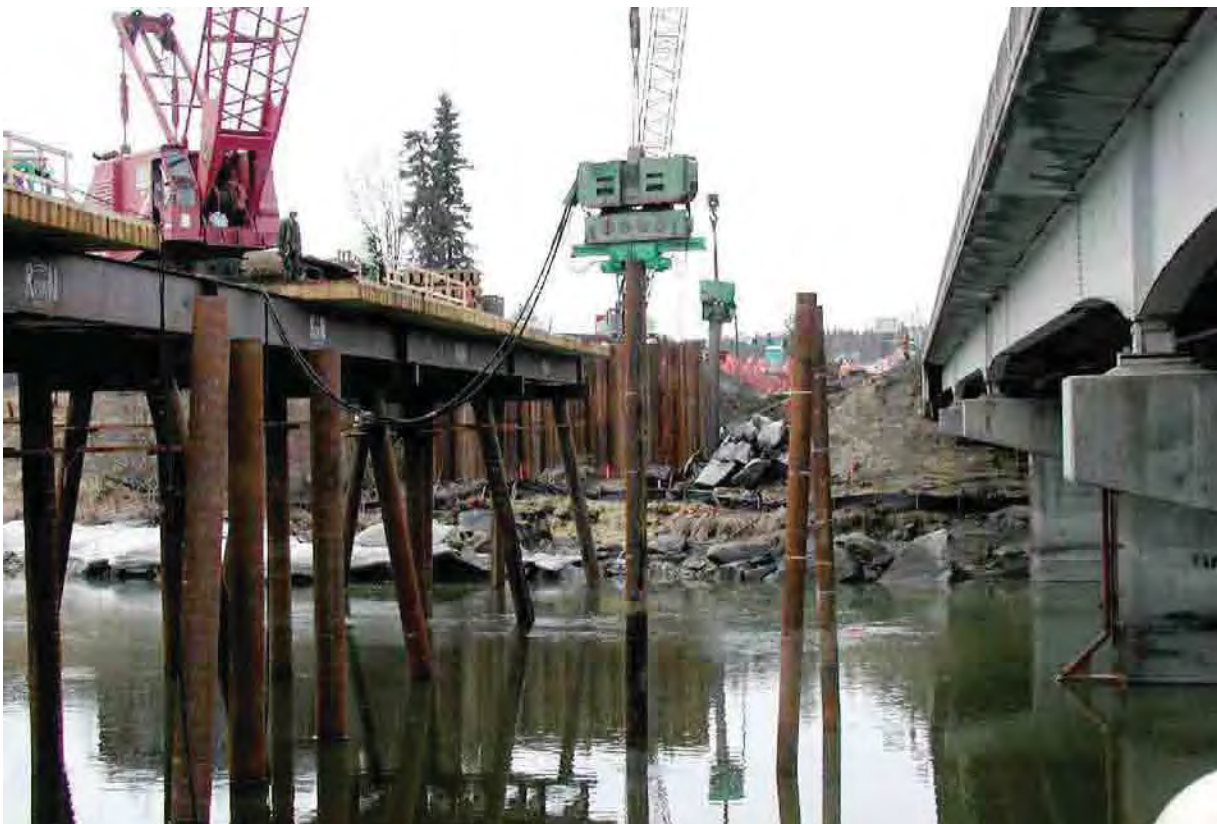
Figure 4 - Temporary trestle style work/detour bridge (Soldotna, AK)
