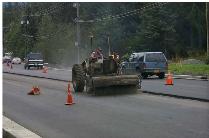
Figure 4-2 Surface Preparation before Applying Tack
