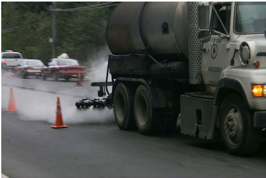
Figure 4-1 Spraying Tack Coat
