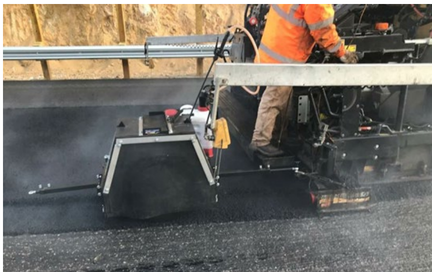
Figure 7-3 Step Taper Shoe With Compactor
