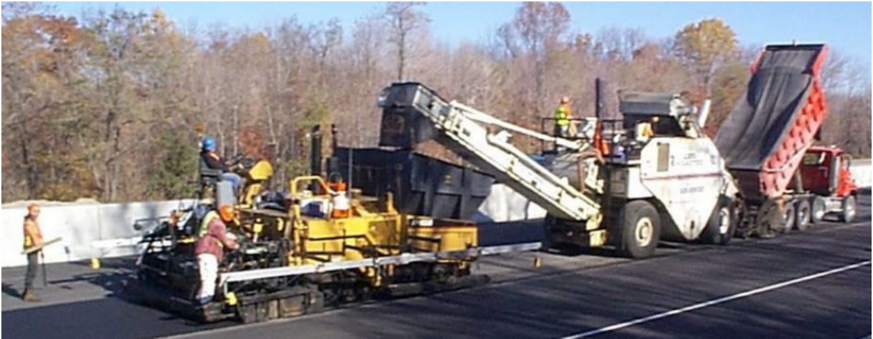
Figure 7-5 Pickup Machine Feeding Paver
