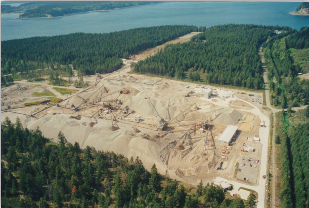
FIGURE 9 CALPORTLAND PIONEER AGGREGATE PLANT
