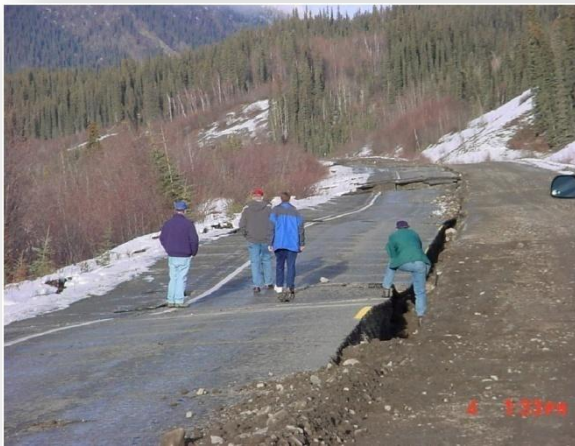
Earthquake damage to Tok Cutoff Highway, 2002
