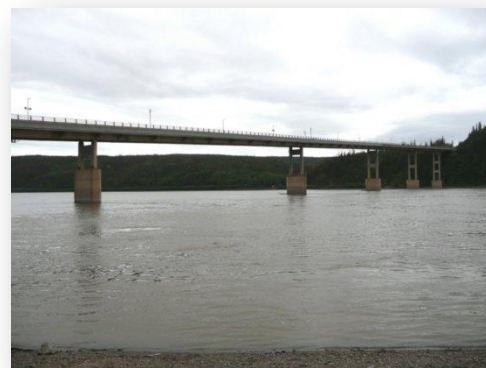
Yukon River Bridge
